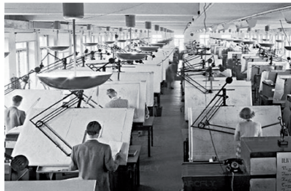
Fig. 1. Former Design Offices
