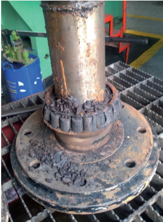
Fig. 2. Upper bearing of the jib crane bracket.
